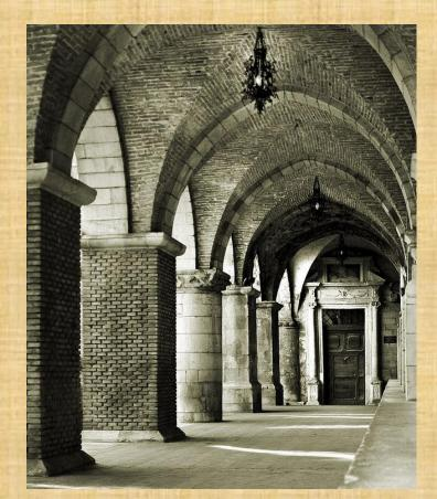
cross vault = double barrel vault = groin vault
